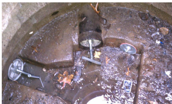
Photos of the manhole outside of the Calf Pasture Beach concession stand. The green substance is the result of a dye test which proved that the concession stand was connected to the storm drain system and not the sewer (Above). After the smoke test showed that all drains in the concession stand we're connected to the storm drain system, they we're plugged to prevent any further leaking before the lines were rerouted (Right).
