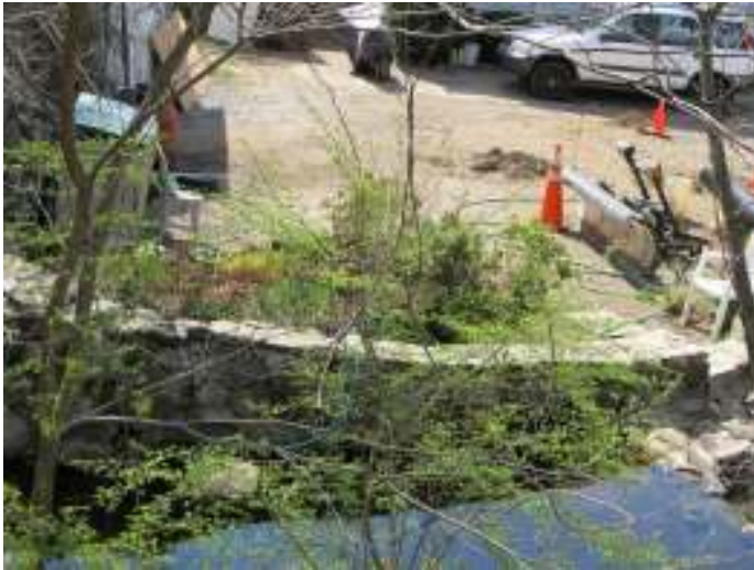
Suspected percolation test for replacing the cesspool at house number 64. Photo taken on 4/10/12.
